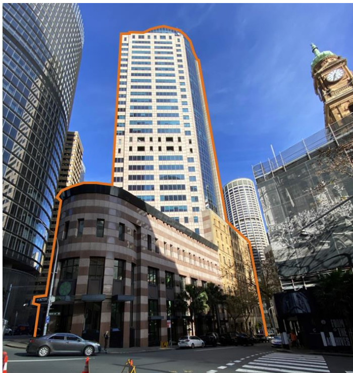
Figure 3: View south-west to the site along Bent Street towards Spring Street
